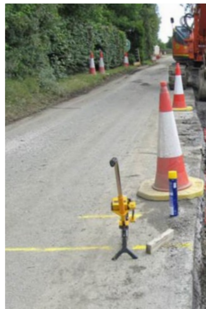
Onshore Cable Installation
